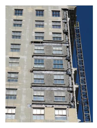
Figure 5: Corner and wall field repairs conducted on both the northeast and southeast corners. Steel repairs, brick replacement, waterproofing, new lintels, new sills were installed.
