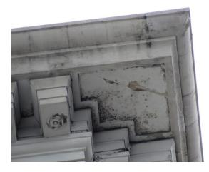
Figure 4: 6 ft fracture along corner cornice stone.
