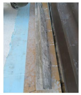
Figure 1:Discovered failing patch at cornice edge 19 stories high (left). Failed patches removed during the inspection identified helical ties had been used to fasten the new patches to the parent stone (right).
