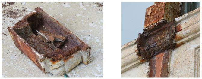
Figure 2: Cast iron window mullion piece discovered on a setback. This led to a full survey and repair campaign of the entire facade.
