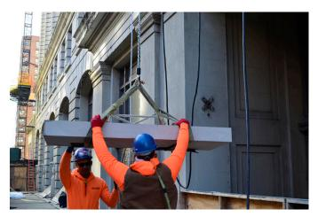
Figure 8: Installation of a stone lintel in progress
