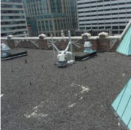
Top left, bottom left: Roof prior to replacement. Top right and bottom center: roof after replacement. Bottom right: restored bulkhead.
