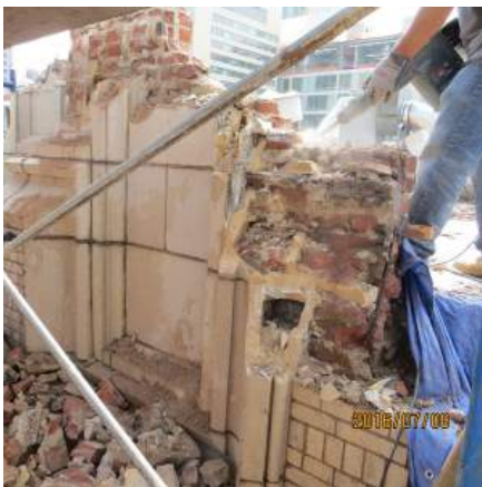
Above: Detail drawing of pre-cast concrete unit for parapet. Top left, and bottom left, center and right: during demolition and construction of parapet. Top right: Portion of restored parapet and coping.
