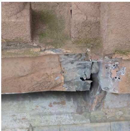
Top left: Sandstone around window before restoration. Top right, bottom left, right and center: Restored sandstone.
