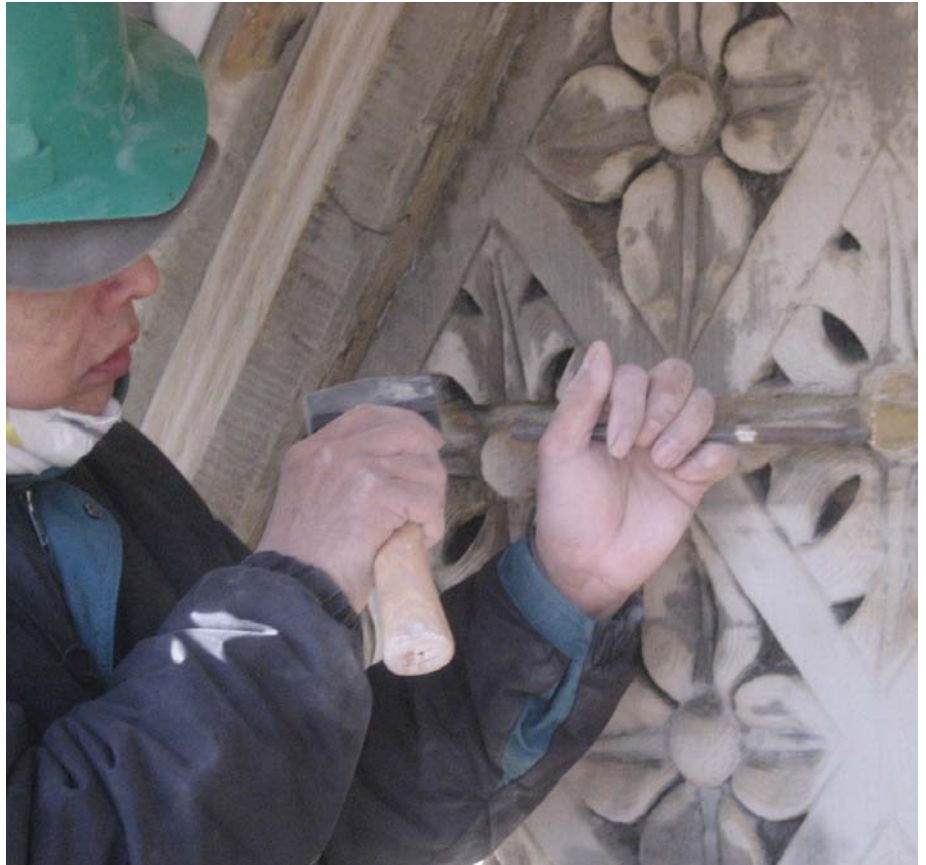
Top left: Deteriorated stone before restoration. Bottom left: Stone ornament after re-carving. Top right: Re-carving stone in place. Bottom center: Deteriorated stone before. Bottom right: Newly carved stone ornament replaces highly eroded original carving.
