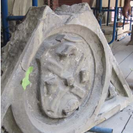
Top left: Worn sandstone gable ornament before. Top right: Replacement sandstone gable ornament. Bottom left: Matching tooled sandstone. Bottom center: Sandstone ornament before. Bottom left: Sandstone ornament after.
