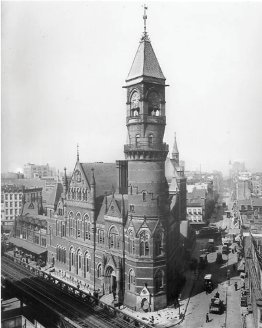
Jefferson Market Courthouse in the early 1900s (from the National Park Service Office of Archeology and Historic Preservation's Historic American Buildings Survey of 1968)
