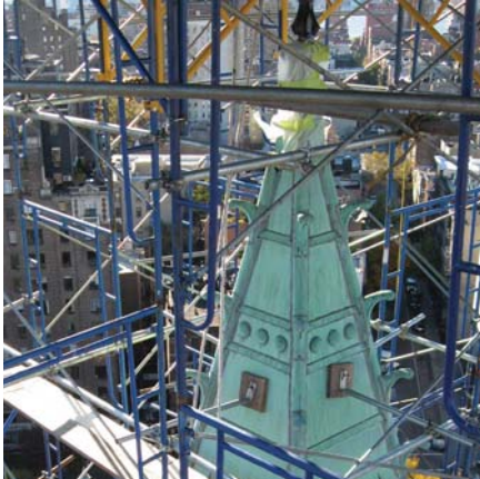
Top left: Tower cap during restoration. Top right: Scaffolding allowing work to be done on tower cap and finial. Bottom left and center: Newly fabricated copper finial on tower cap during restoration. Bottom left: Interior of tower cap.
