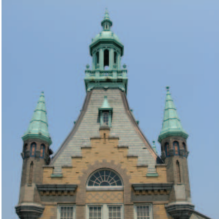
Top, left: Tower before restoration. Top, right: Tower after restoration. Bottom: Turret roof after restoration.
