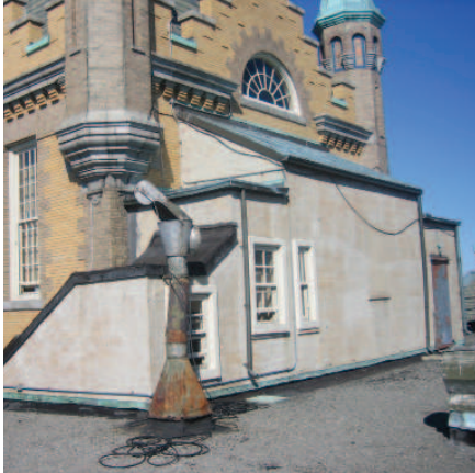
Top, left: Bulkhead before restoration. Top, right: Bulkhead after restoration. Bottom, left: New railing installed on roof. Bottom, center: Inferior workmanship discovered inside existing parapet. Bottom, right: New parapets on 1950s wing after restoration.
