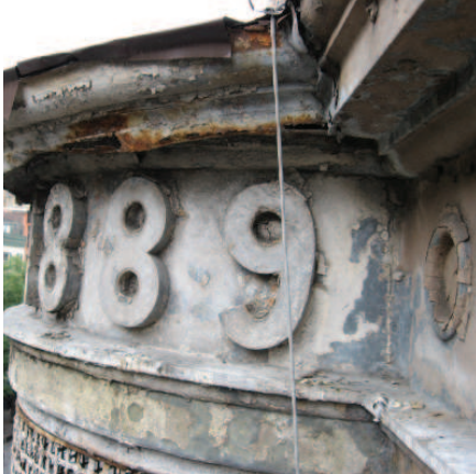
Top, left: Ornamental sheet metal before restoration. Top, right: Ornamental sheet metal, after restoration. Bottom, left: Lintel above 4th floor columns, before restoration. Bottom, center: Lintel above 4th floor columns, after restoration. Bottom, right: New cornice installed.
