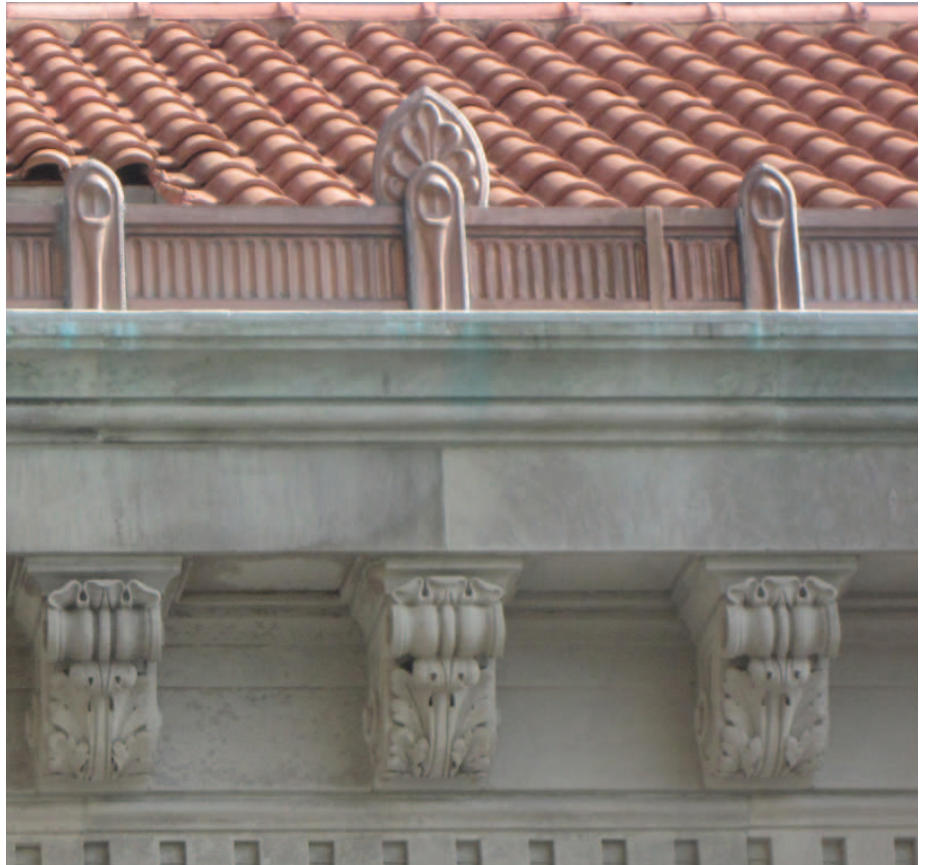
Top, left: Parapet shown before copper cresting was installed. Bottom, left: Old gutter system. Bottom, center: Clay mockup for copper cresting. Bottom, right: New copper cresting and gutter viewed from roof. Top, right: Copper cresting installed atop parapet.
