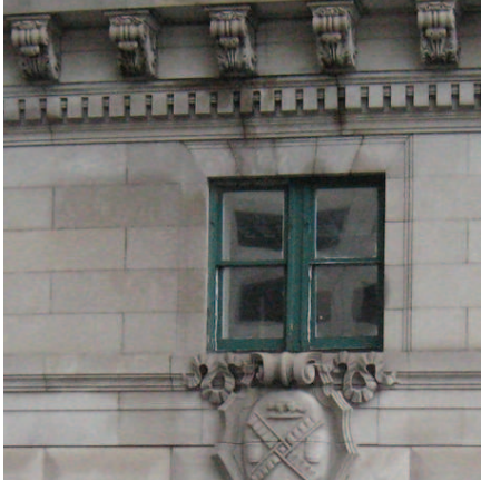
Top, left: Masonry stained by leakage from above. Bottom, left: biological growth on masonry. Bottom, right: Thin joints between stone required careful use of hand tools for pointing work. Top, right: Masonry after restoration.
