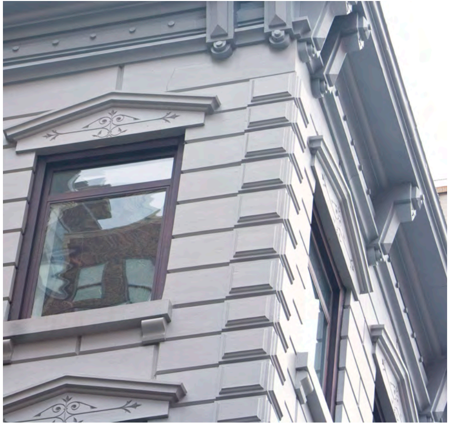
Top and bottom left, bottom center: Cast iron before restoration. Top right: Cast-iron clad facade after repair. Bottom right: Test units during restoration.
