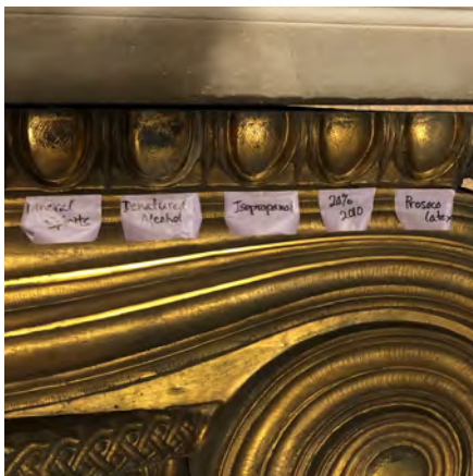
Top left: Cleaning mock-up at plated bronze; Bottom left: Plated bronze capital before cleaning; Bottom middle: limestone before repair; Top left; base of limestone pilaster af- ter restoration; Bottom right: Gilded limestone column capital after cleaning
