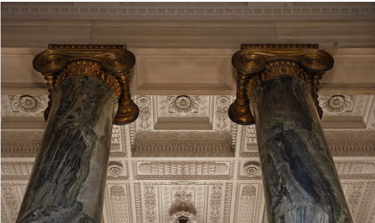
Plaster ceiling, marble columns with bronze capitals, after restoration. Photo: Whitney Cox
