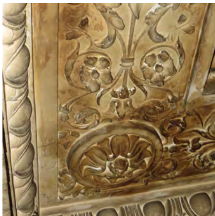
Top, middle, and bottom left: Staining and efflorescence in plaster ceiling due to water penetration; Top right: Ceilings after restoration; Bottom middle: Primed ceiling before painting; Bottom right: ceiling restoration in progress.
