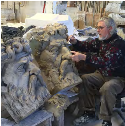
Above: Terra cotta before restoration; Left middle: Sculptor at Gladding McBean carves replica of terra cotta sculpture as replacement; Bottom row and top right: Terra cotta after restoration.
