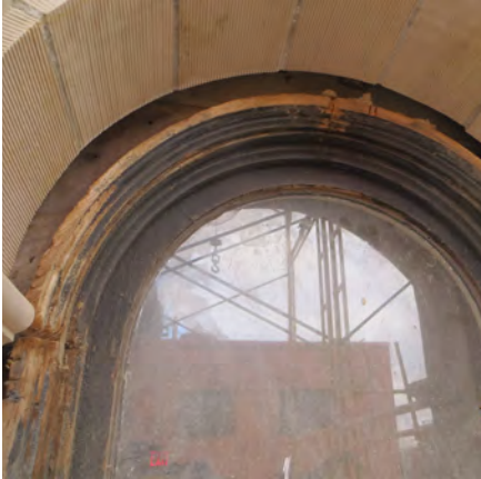
Top left: Head condition—Deteriorated wood frame and missing brickmold on window type W2; Bottom left: Jamb condition—deteriorated wood frame and the transom, window type W1; Bottom center: Jamb condition—deteriorated wood frame and mullion; WIndow type W13; Top and bottom right: Newly installed windows.
