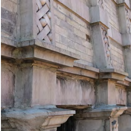
Top, middle and bottom left: Terra cotta before restoration; Bottom middle: extensive facade deterioration resulting in vegetation growing on the building; Top and bottom right: terra cotta after restoration
