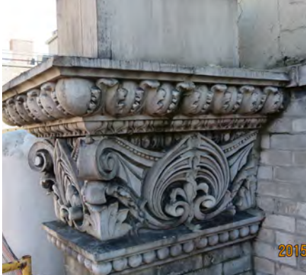
Above: Terra cotta before restoration; Left middle: Sculptor at Gladding McBean carves replica of terra cotta sculpture as replacement; Bottom row and top right: Terra cotta after restoration.
